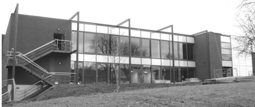
Figure 3: The Keith Green Building under construction; December 2005
